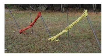
Take a short steel rod for use as a spinner rod (minimum 2' by 3/8" diameter), and put it through the turns of the lashing rope, twisting until the lashing is tight, and then drive the short picket into the ground.
