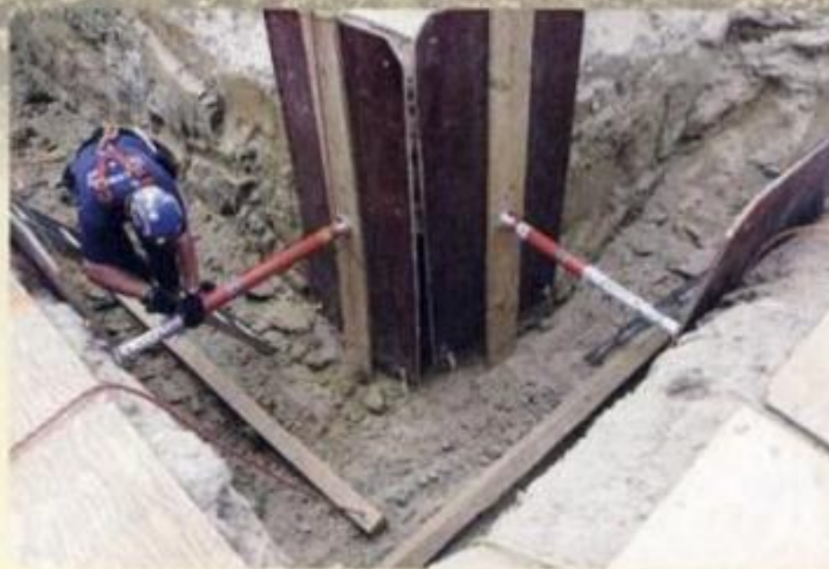
2 The first set of panels is installed on the inside L corners with middle shore shot.
