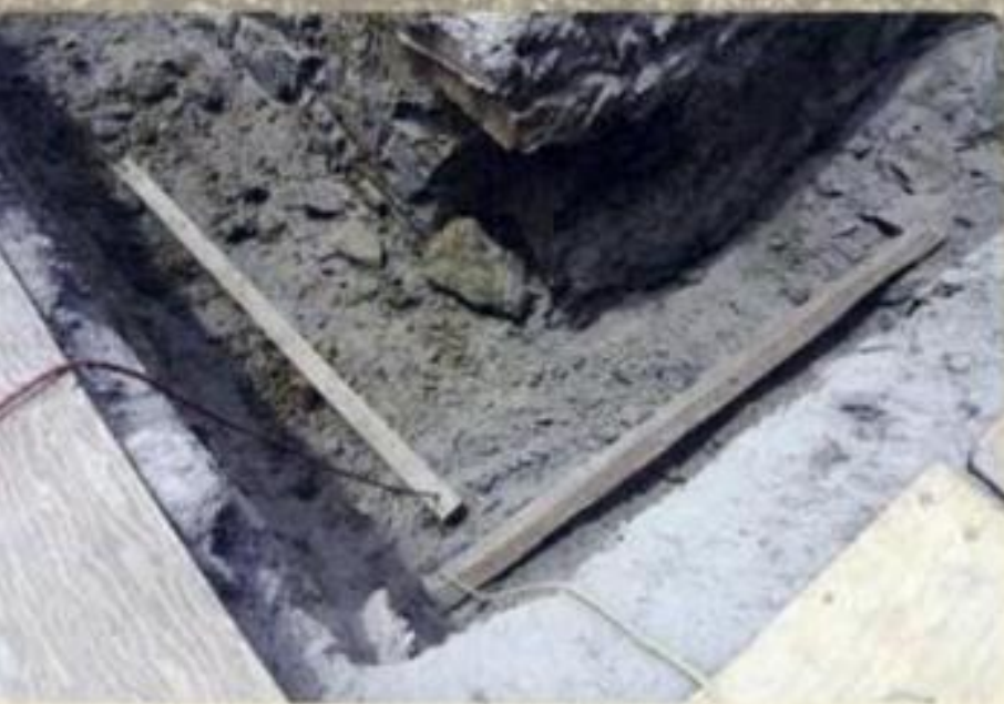
1 Wales are placed in the bottom of trench.
