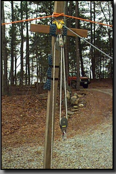
Square lashing is used to hold two timbers together that cross at right angles.
