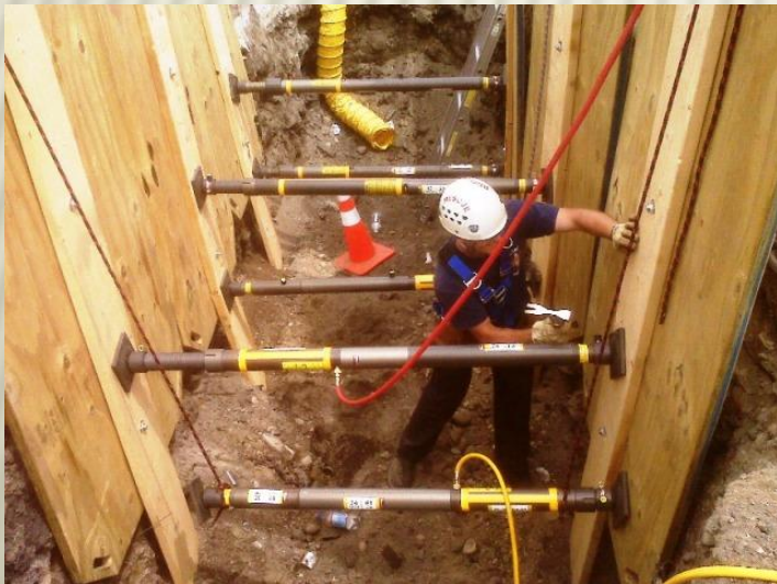
Trench Rescue Struts
